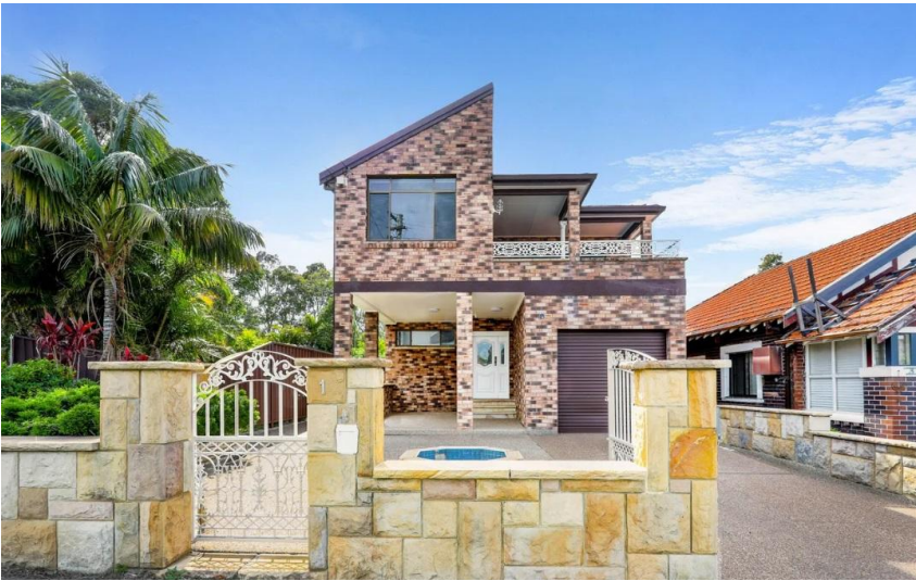
view 01 - 1 KING ST FRONT FACADE
