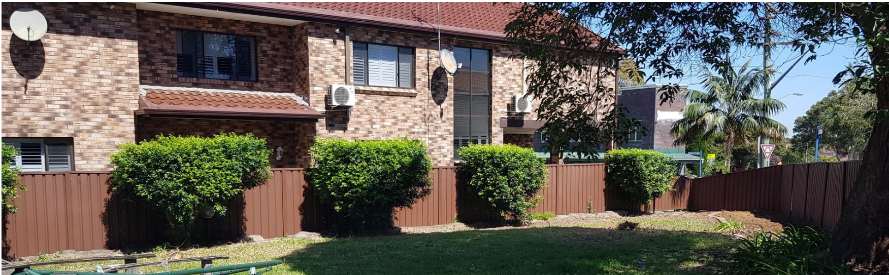
1 KING ST - existing side facade from site
